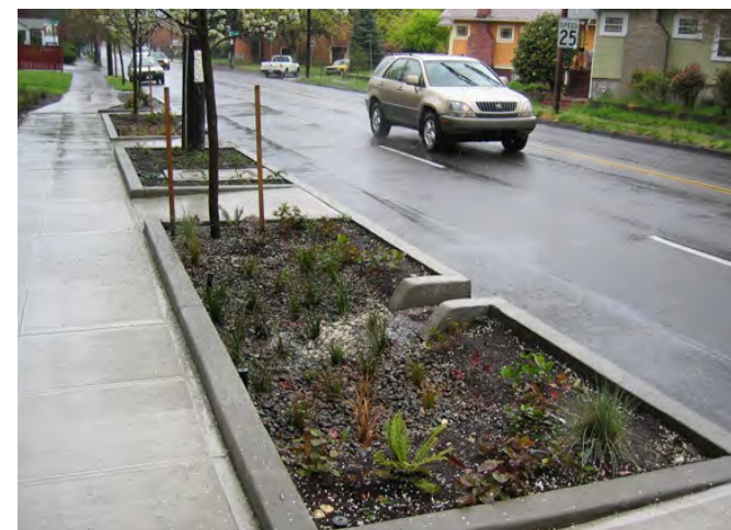
Rain garden with pebbles and plants creates permeable surface, absorbing and filtering rain water from street during storm.
