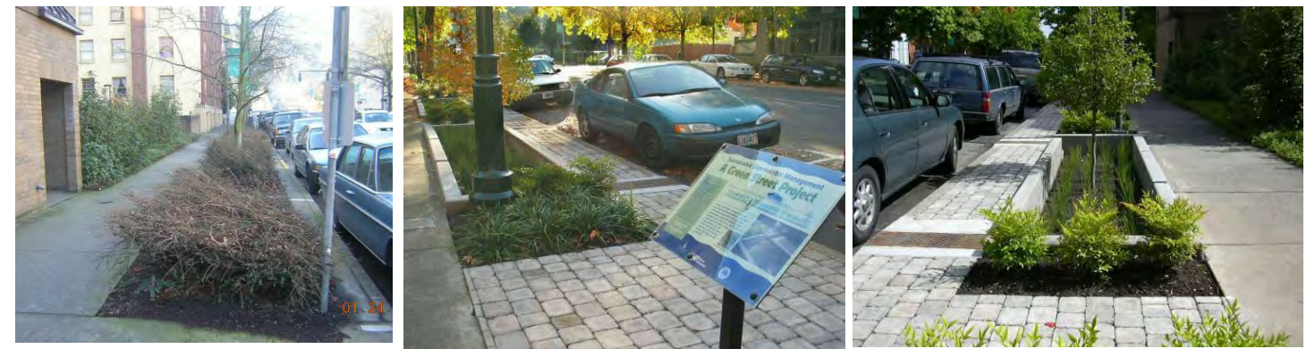
Portland "green street" before and after with rain garden, grate, and permeable bricks to collect and divert stormwater.
