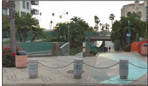
Image 27. Oceanside Pedestrian Tunnel
