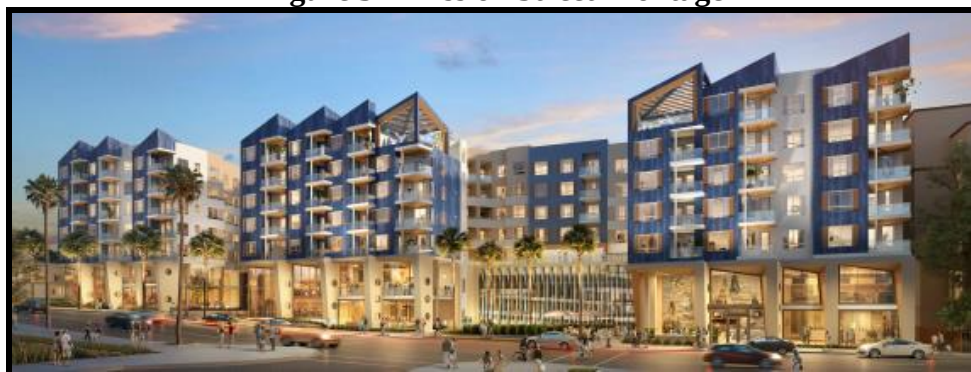
Figure 3 – Mission Street Frontage
