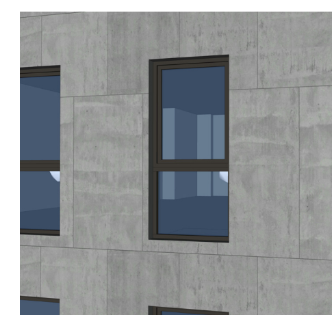
17. BOARD FORM CONCRETE PANELS
