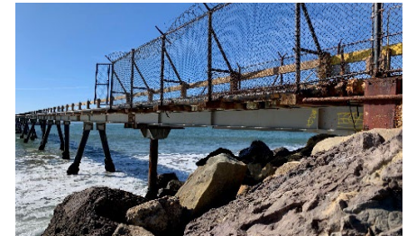
Photo 4: Rincon Pier Structural Assessment
