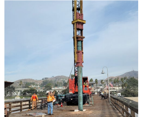
Photo 4: Ventura Pier Storm Damage Repair
