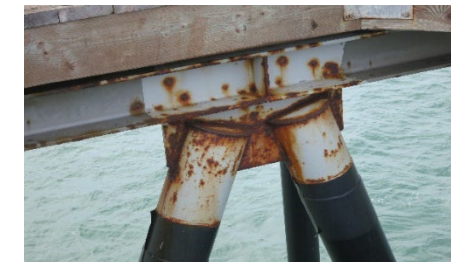
Photo 4: Ventura Pier Corrosion Repair Project
