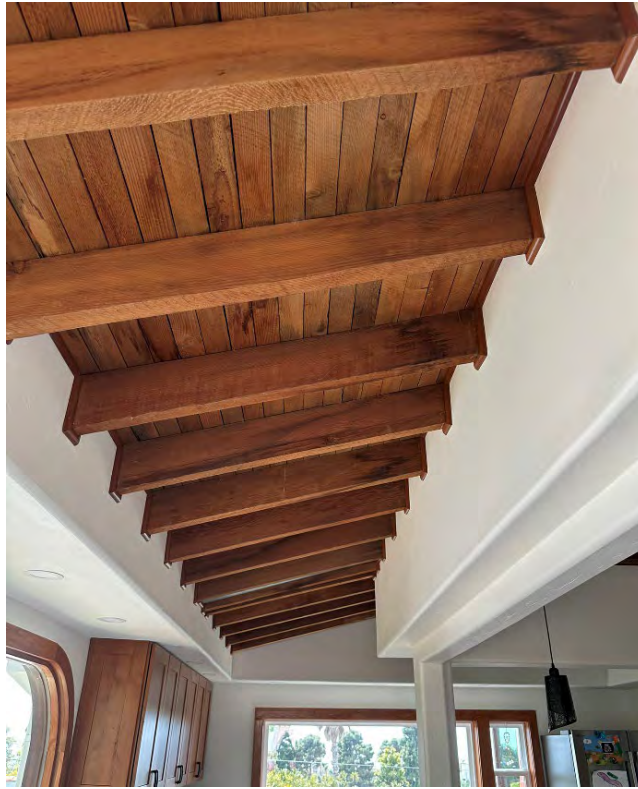
Above: Exposed beams in original shed porch (now enclosed)
