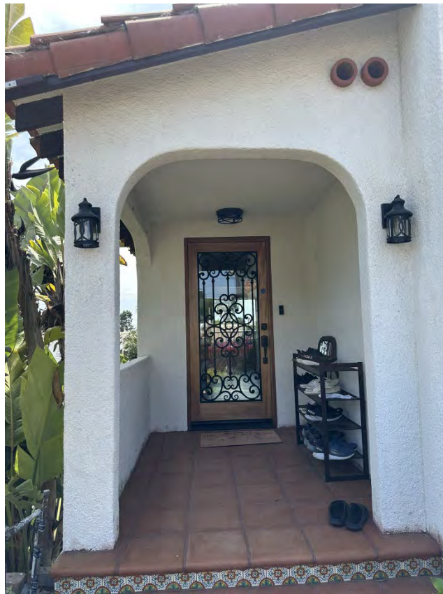
Below: Porch and entry way
