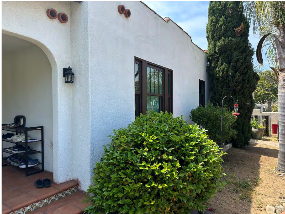
Below: East elevation looking northerly
