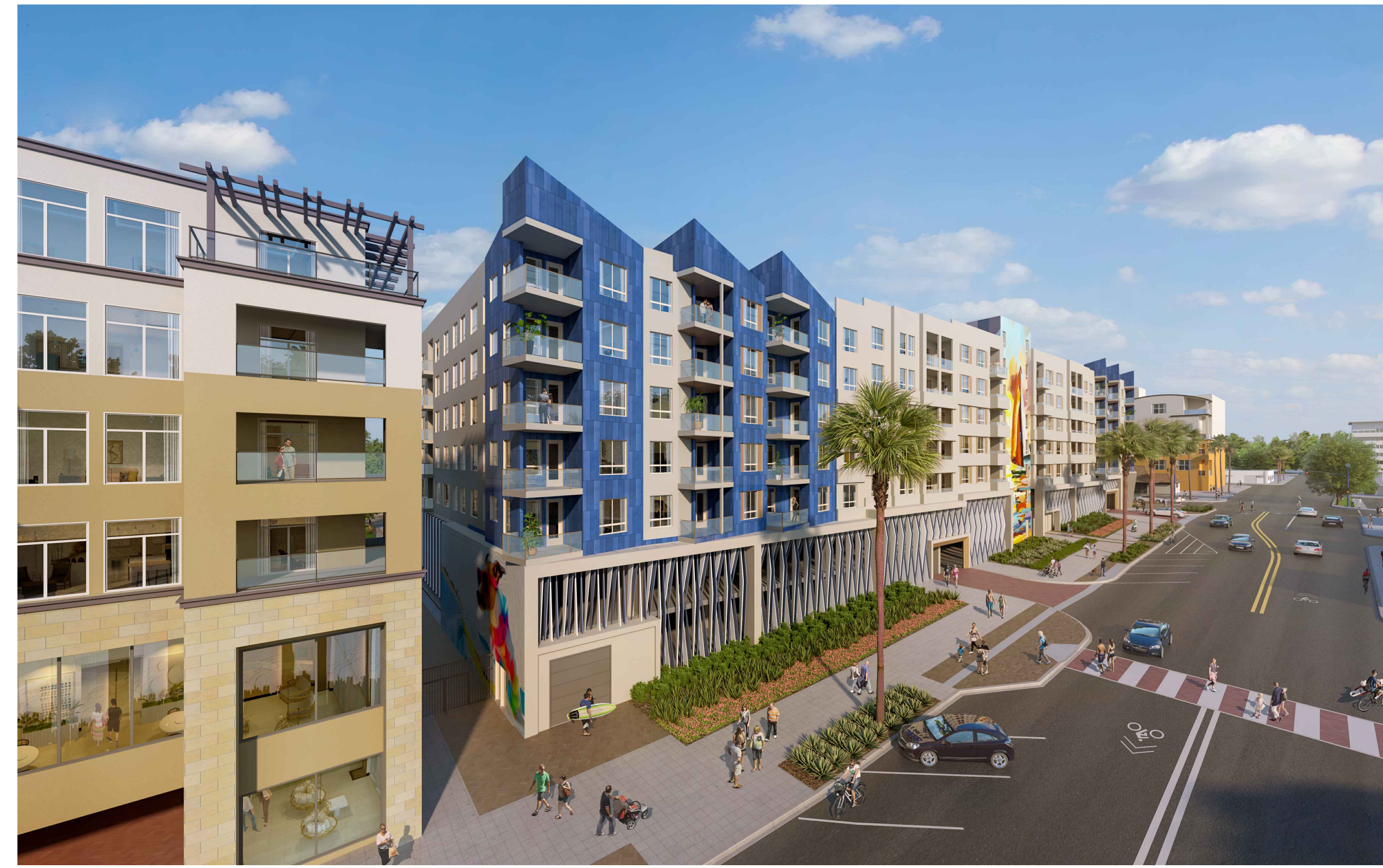
VIEW ON SEAGAZE DRIVE LOOKING NORTHEAST 6
