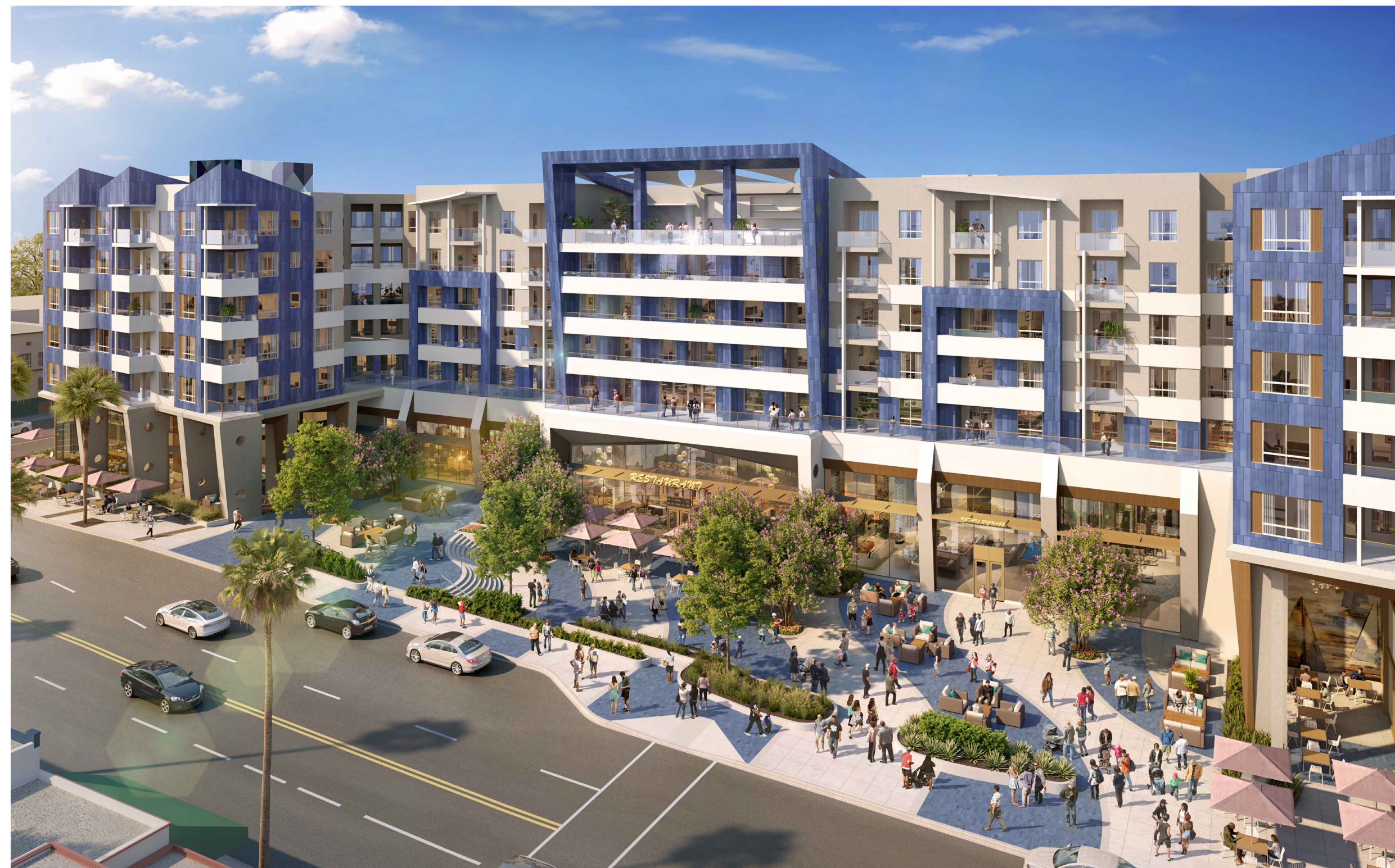
VIEW OF PLAZA ON MISSION AVE LOOKING EAST 5
