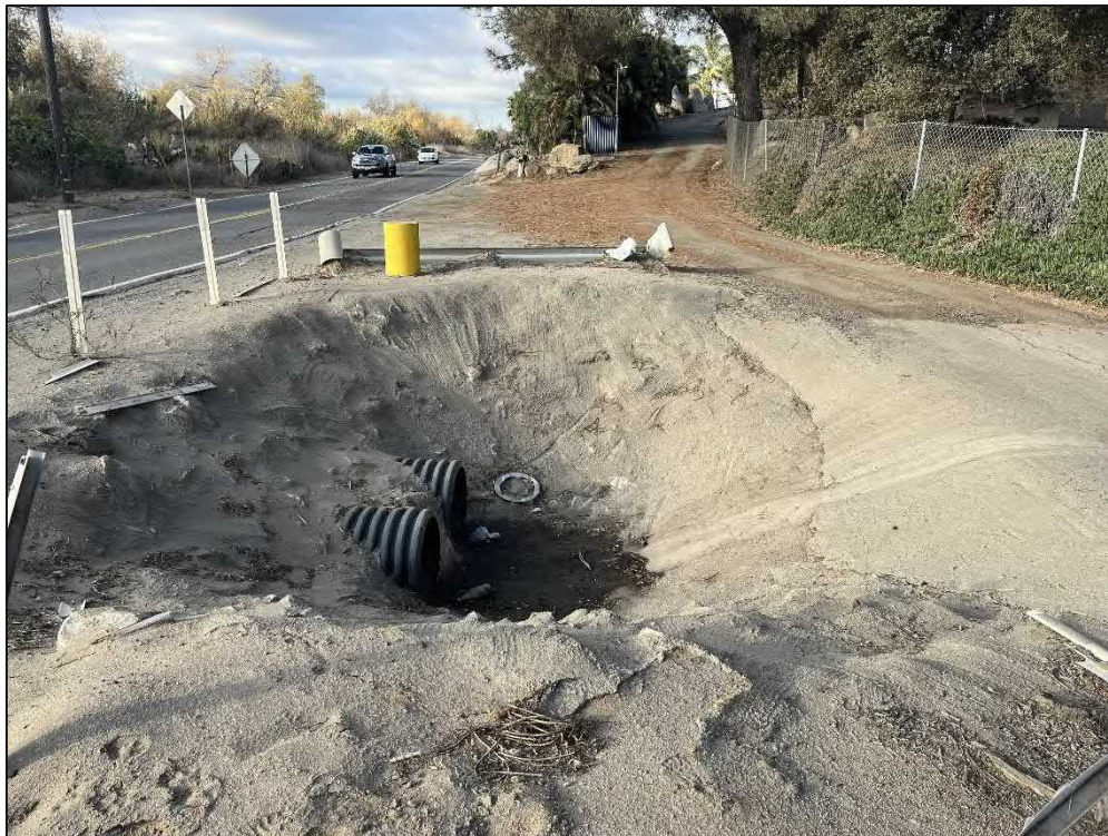
Exhibit 2. Overview of Culvert 3, view facing west.
