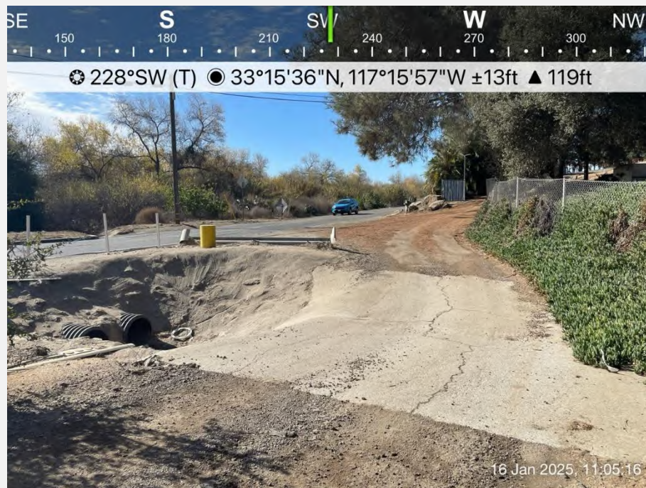
Photo 7. NWW-02 flow path over Arizona crossing and into culverts under North River Road (Photo Point 5).
