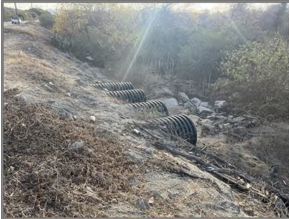
Exhibit 1. Overview of Culvert 2, view facing east.
