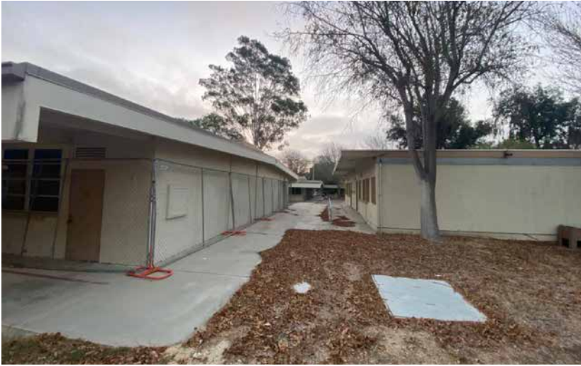
View east towards typical classroom and staff lounge/library building
