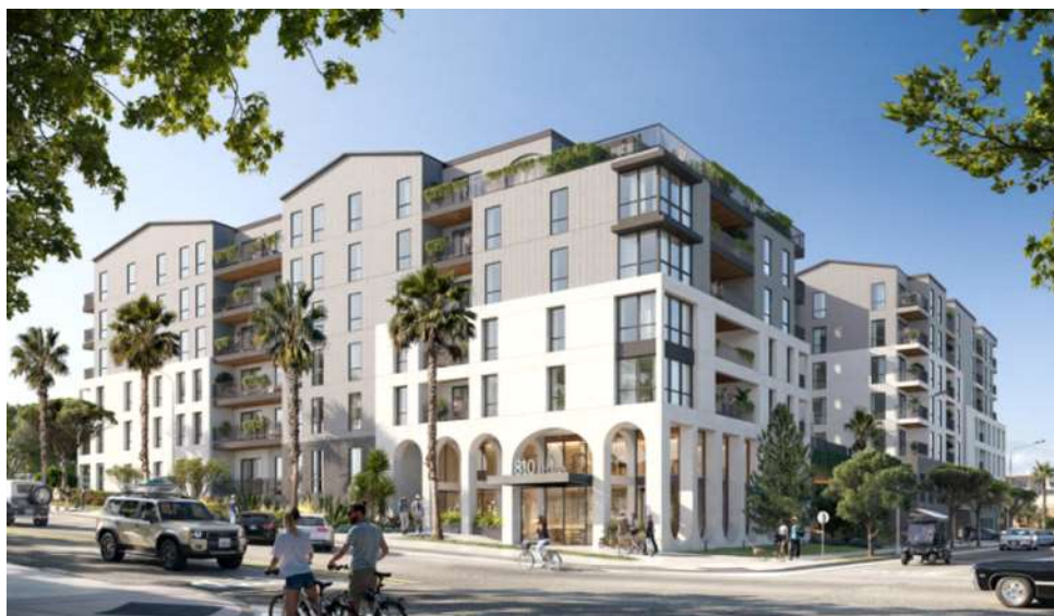
Figure 3 - Mission Street Frontage
